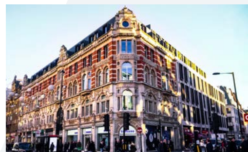
工商大廈 Industrial and Commercial Buildings
